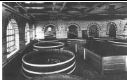
Decorative glazed brickwork in the fermenting room of the Mersey Brewery, Liverpool Photo: Whitbread Archives
